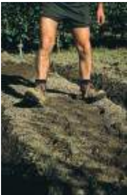
Compacting soil removes any air pockets.
